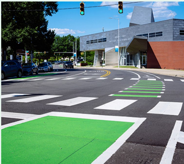
Figure 25: 10th Ave S Bike lanes
